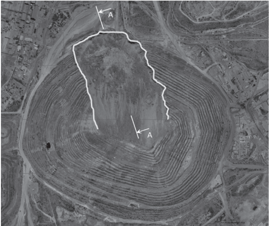
Fig. 14 - Plan view of North Wall failure at Palabora mine
